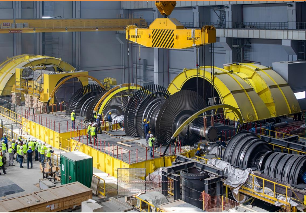
Installation of the Arabelle turbine at the first unit of the Akkuyu nuclear power plant, 2024 Photo: Akkuyu Nükleer
